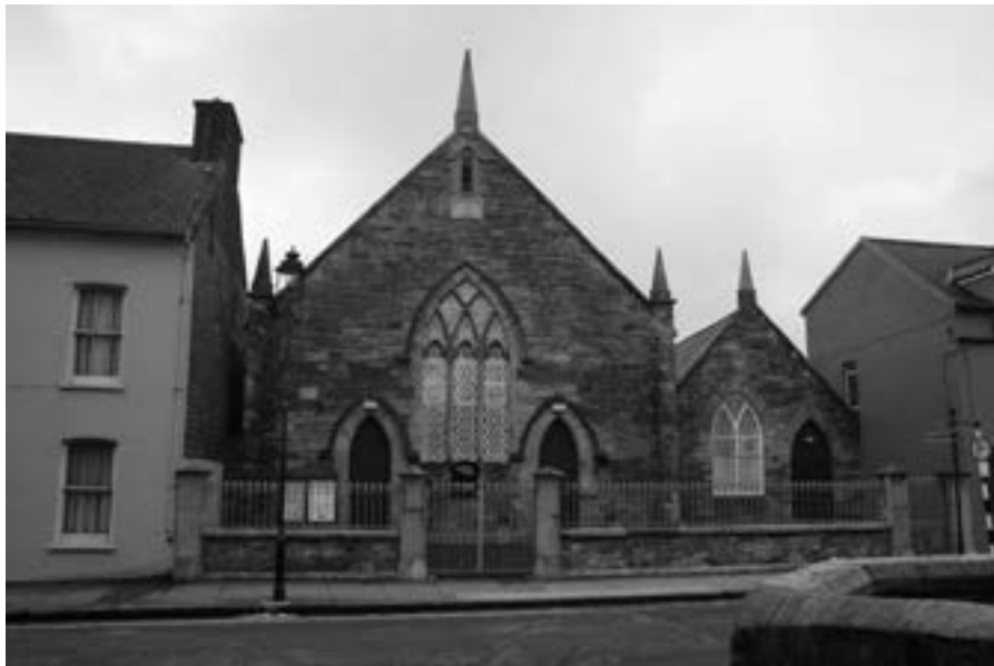
Fig. 15: Methodist church, Kent Street (Photo: author).
