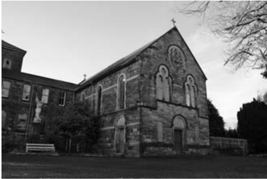
Fig. 22: Convent chapel, viewed from southwest (Photo: Clíodhna O'Leary 2017).
