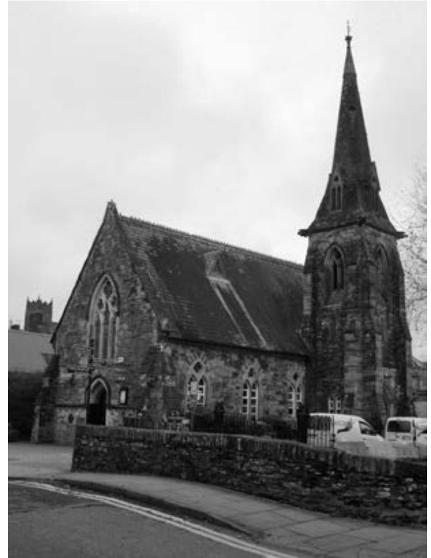
Fig. 19: Former Presbyterian church, viewed from southwest (Photo: author).
