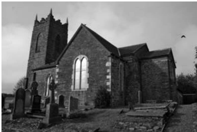
Fig. 10: Kilgarriffe church, viewed from south (Photo: author).
