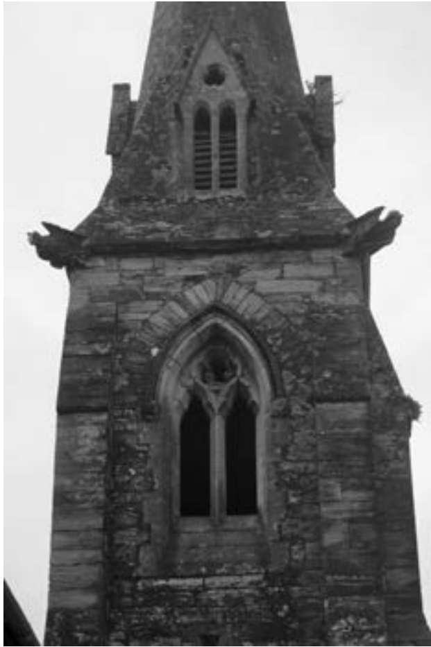
Fig. 20: Tower to Presbyterian church (Photo: author).
